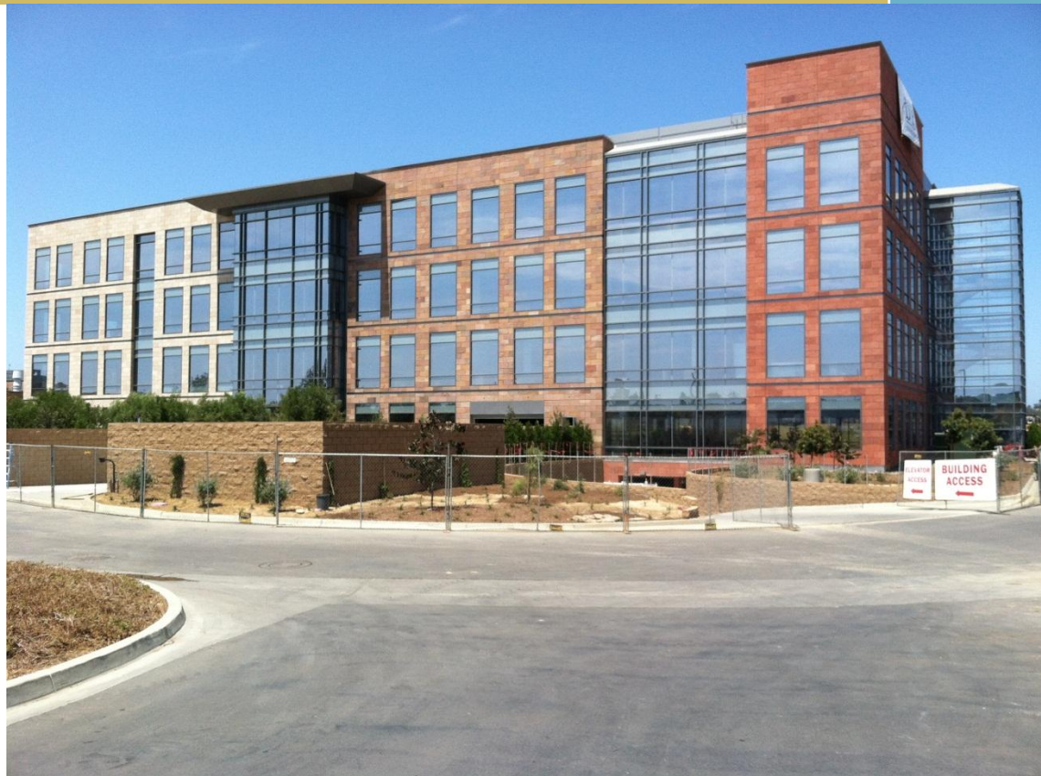
Figure 1: View of Building, Maffett
